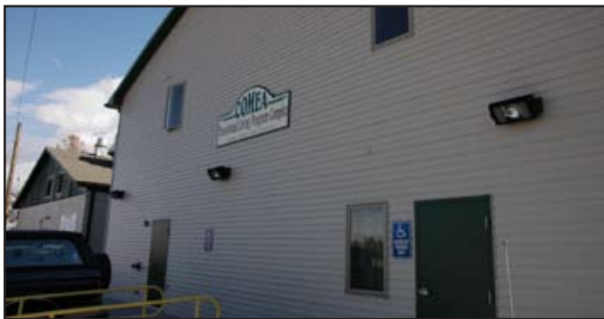
Laramie County received a $200,000 Community Development CDBG for the COMEA (homeless shelter) Transitional Living Units.
