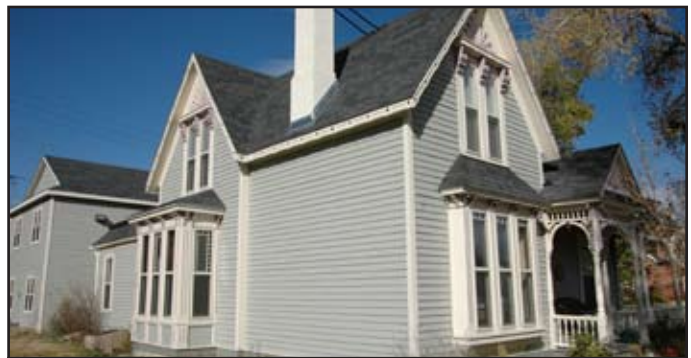
Laramie County received a $250,000 Community Development CDBG for the Wyoming Children’s Society building.
